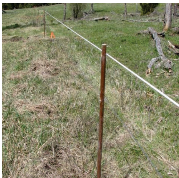
This two-wire seasonal power fence can be used where stock are broken to electric fence. Wooden posts brace the ends. The fiberglass posts can be laid down when the fence is not in use.
